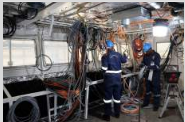
© KSL- Cable dressing in the Bridge for KNS Shupavu of the @KSL- kdfinfo at Mombasa Shipyard. KSL is committed to delivering the vessel within a short time and using minimal resources which will, in the end, go a long way in enhancing safety and security of Kenyans
